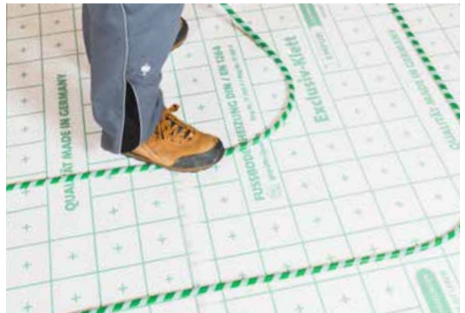
Install the KLIMAPEX® hook and loop pipes using the preprinted laying grid by lightly pressing onto the hook and loop panel.
