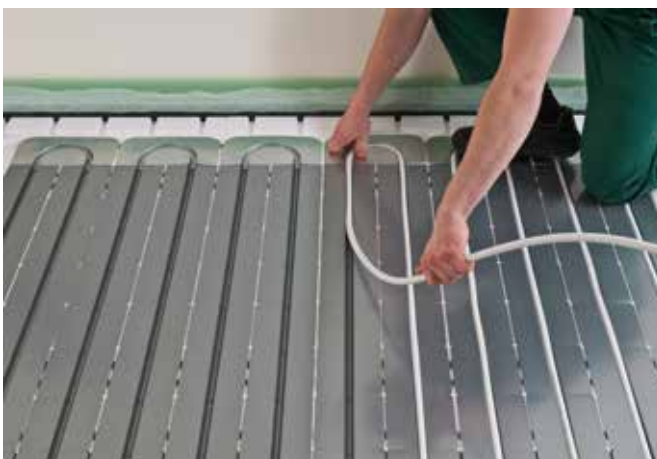
The metal composite pipe is easy to bend and clicks into the sheets with a little pressure.
