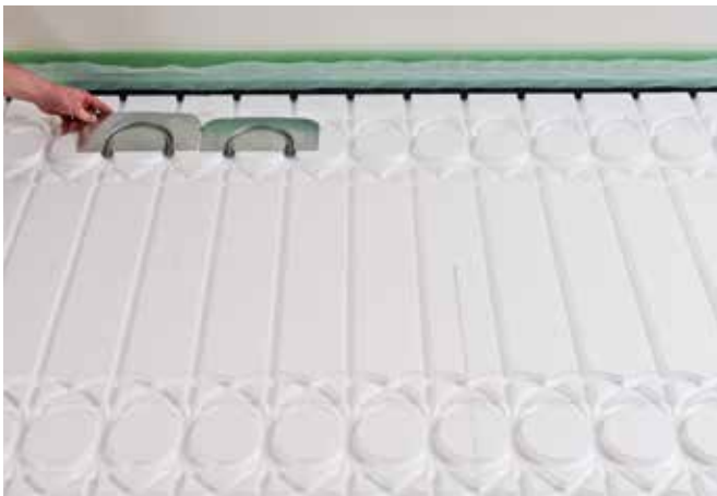
Inserting the aluminium redirection plates into the foamed grooves.
