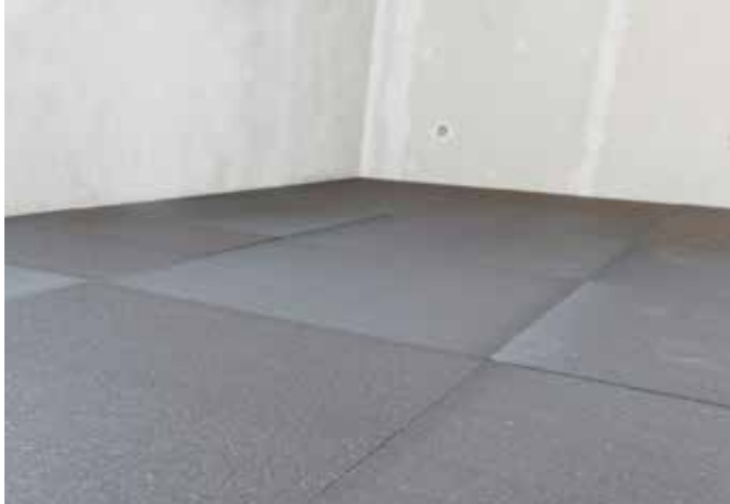
Full-surface laying of the bottom insulation, taking into account the existing supply lines.
